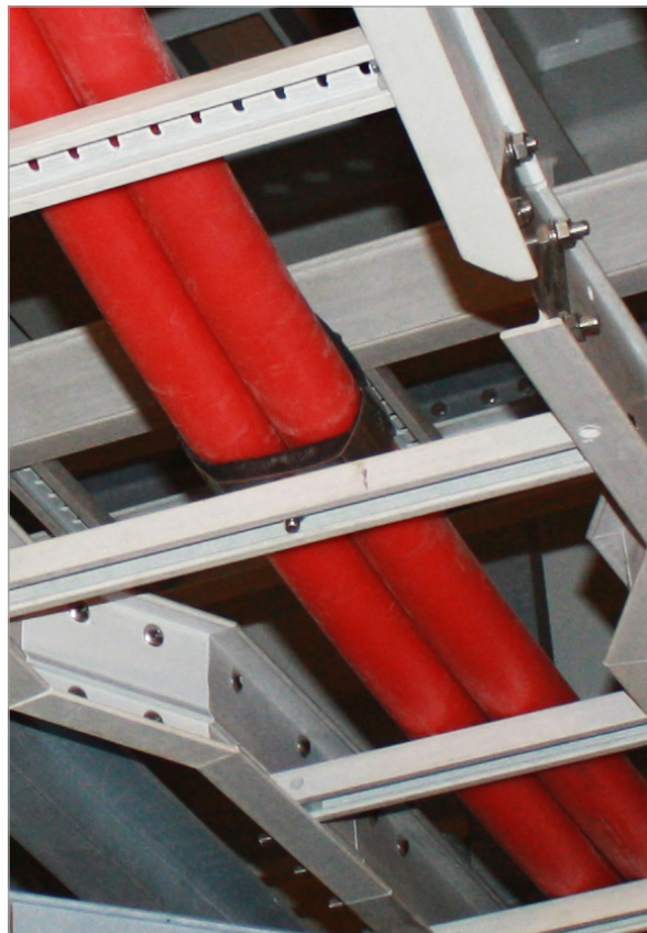
SmartCleat® Trefoil Ø < 39 mm and 39 - 99 mm
