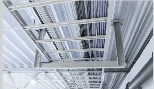
Support channels, Cantilever arms and Ceiling T-supports available in FRP.
